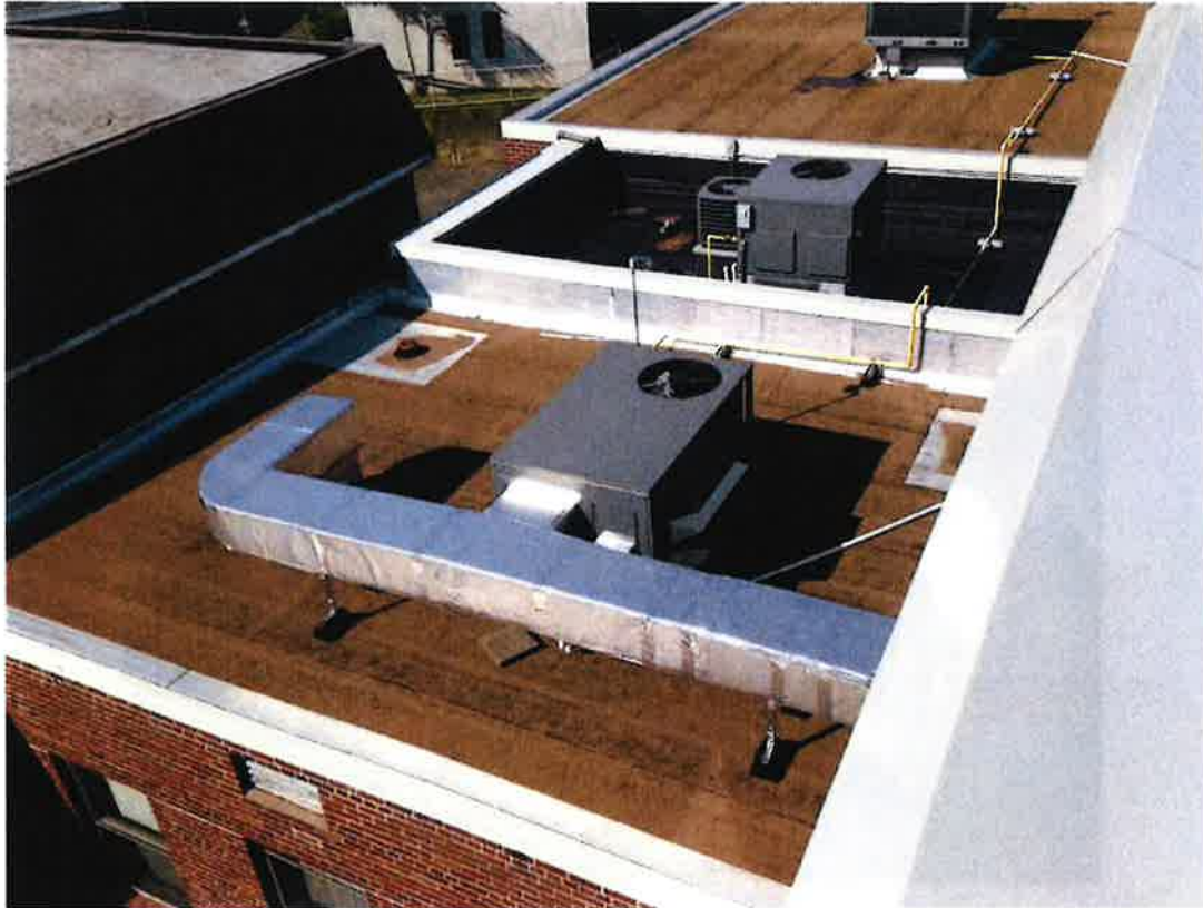
Packaged Rooftop Units and Condensing Unit on Roof
