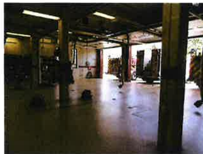
Image 22: Apparatus Bay Clearance Problems
