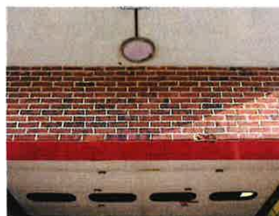
Image 24: Apparatus Bay Door Clearance Problems
