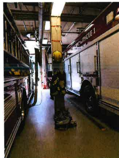
Image 18: Vehicle Exhaust System
