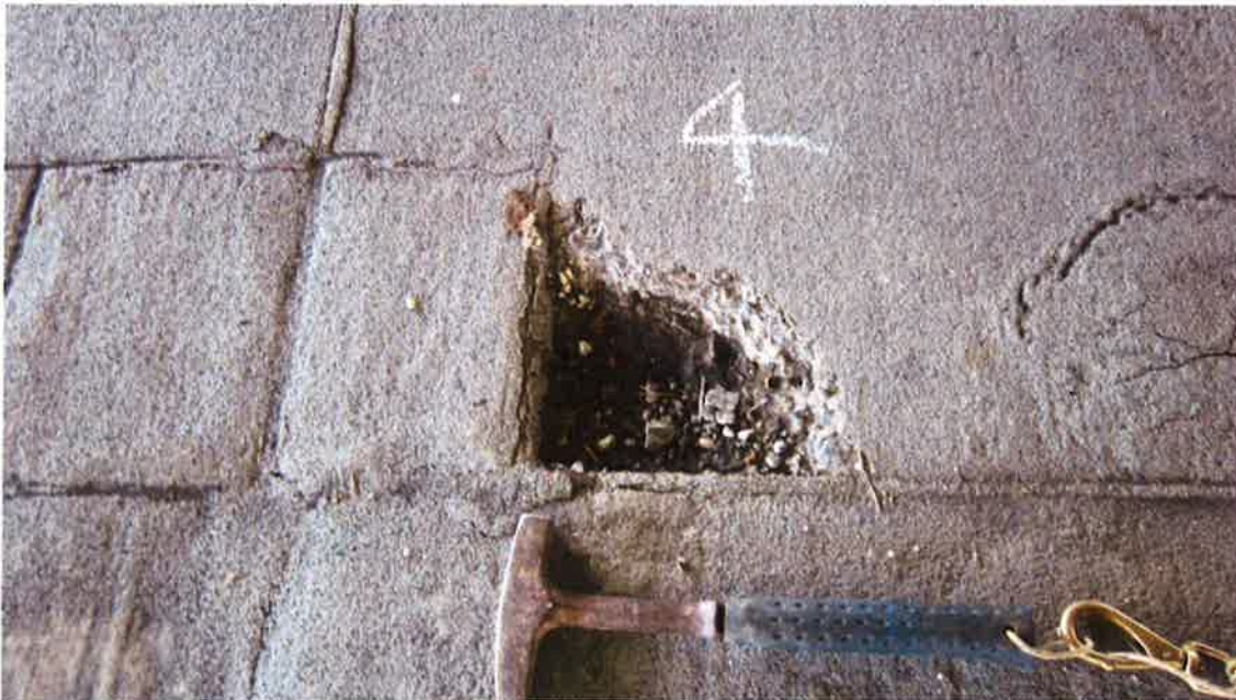
Photo 12- Localized Spall
