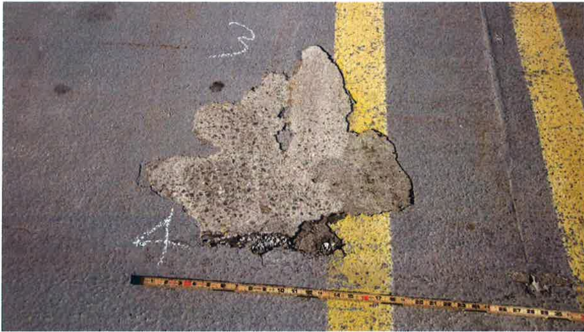
Photo 5- Waterproof Coating Failure
