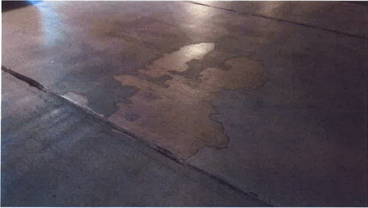
Photo 7- Failed Waterproof Coating
