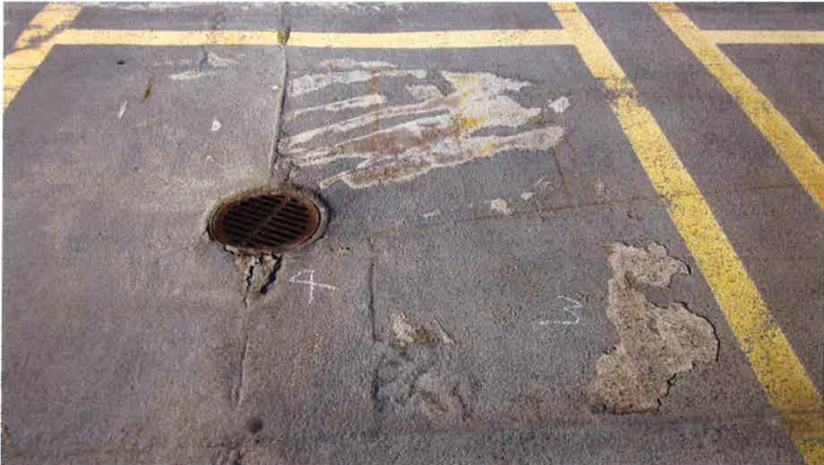
Photo 8- Failed Waterproof Coating and Plow Damage
