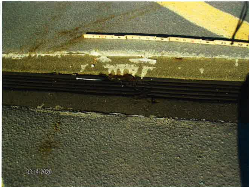
Photo 15- Damaged Expansion Joint
