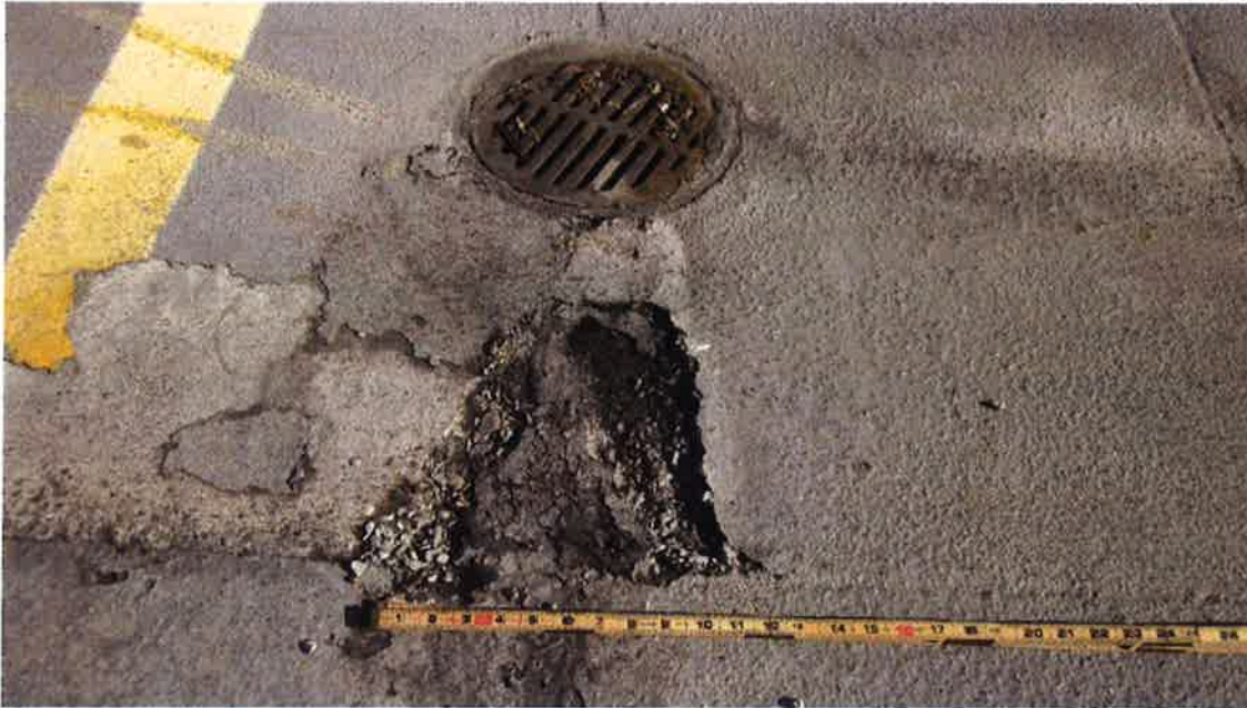
Photo 11- Localized Spall Near Drain
