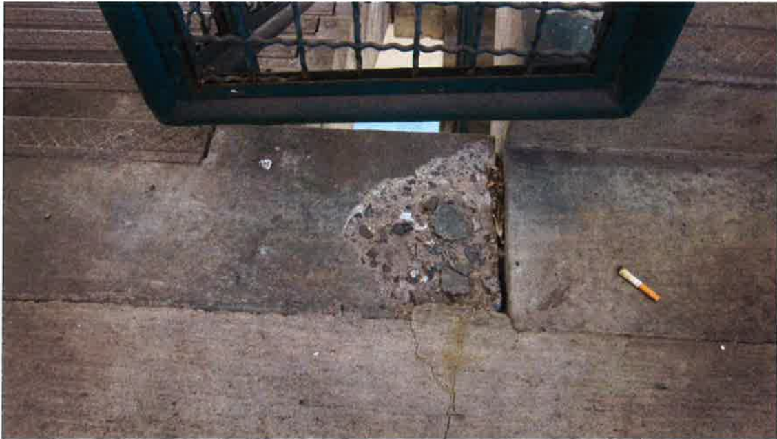
Photo 13- Localized Spall at Stairway Landing
