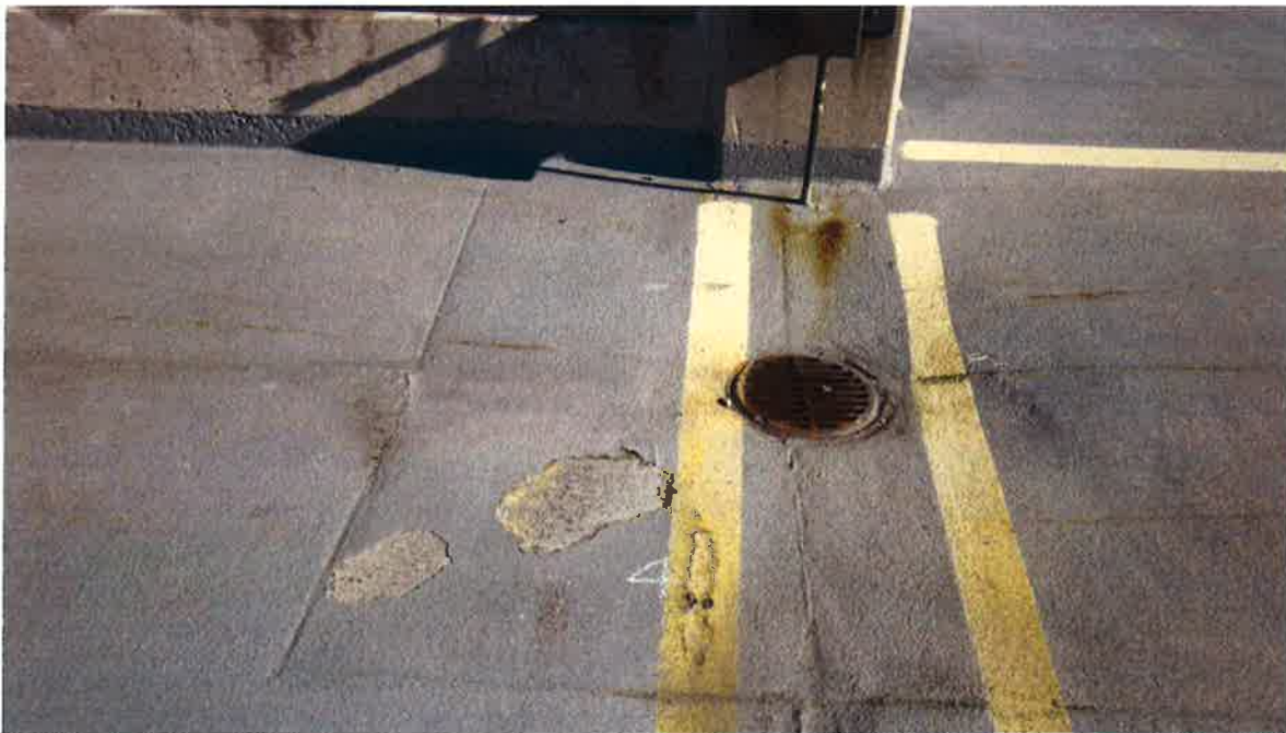
Photo 6- Failed Waterproof Coating
