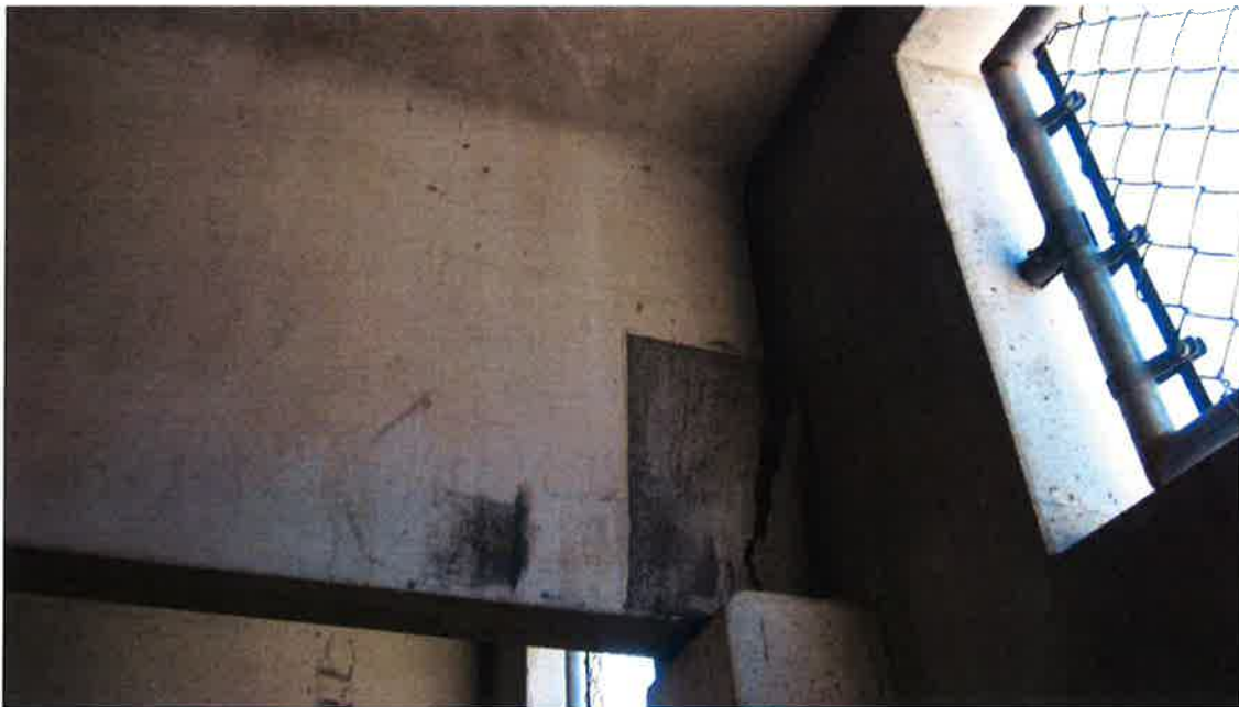
Photo 16- Beam End Spall
