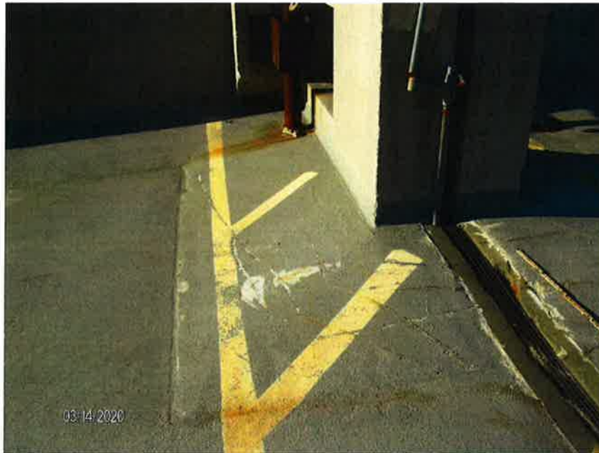
Photo 9- Plow Damage
