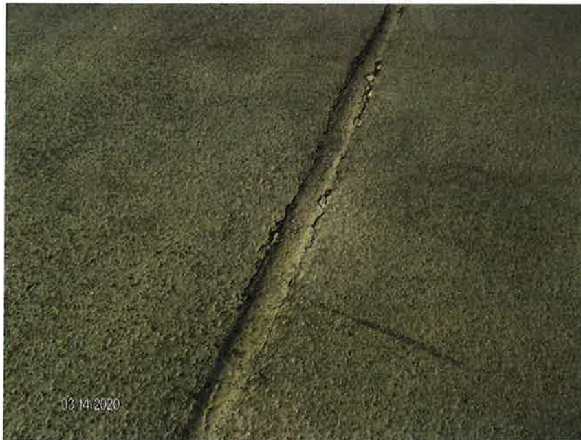
Photo 18- Beam Joint Separation
