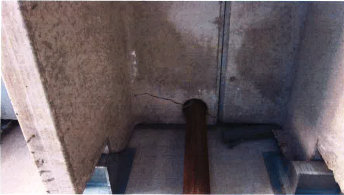
Photo 17- Beam Underside Crack
