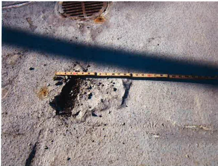
Photo 10- Localized Spall
