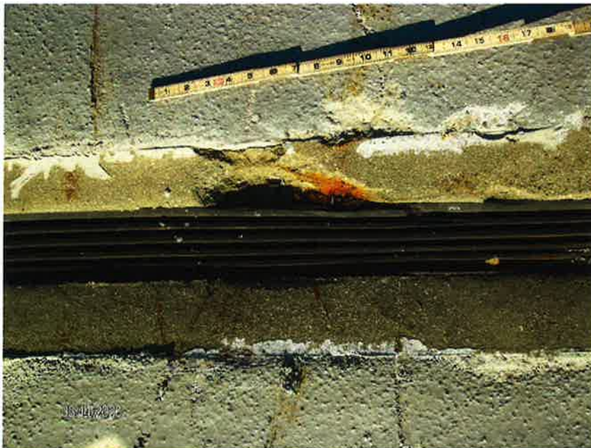
Photo 14- Damaged Expansion Joint
