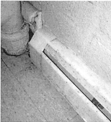
Rusted Base Board Heater
