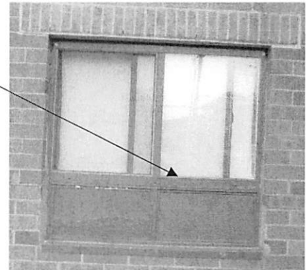
Window damaged, warped and rusted
