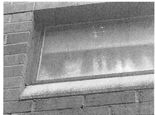
Window with fogged glazing and damaged periphery sealant
