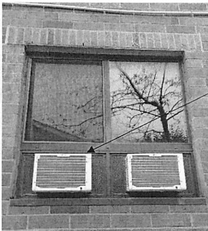
Window Cut for A/C units, and deteriorating periphery sealant.
