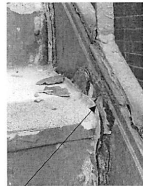
Steel Pans separating from stringer
